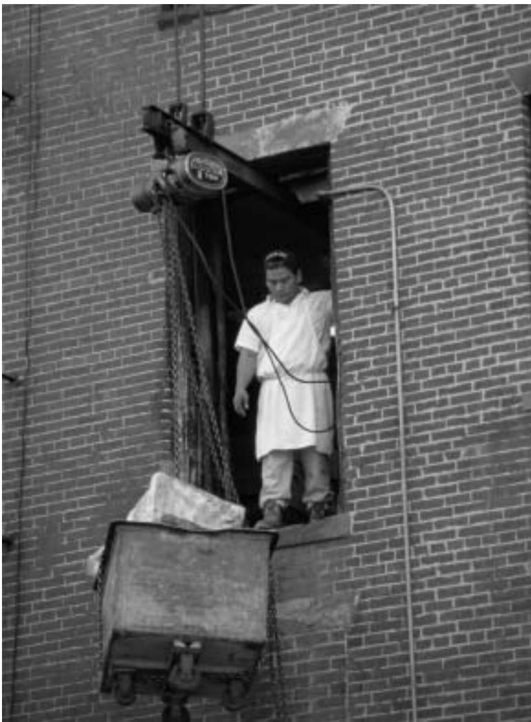
**Figure 1.11** Pulleys make it possible to lift large, heavy loads.
