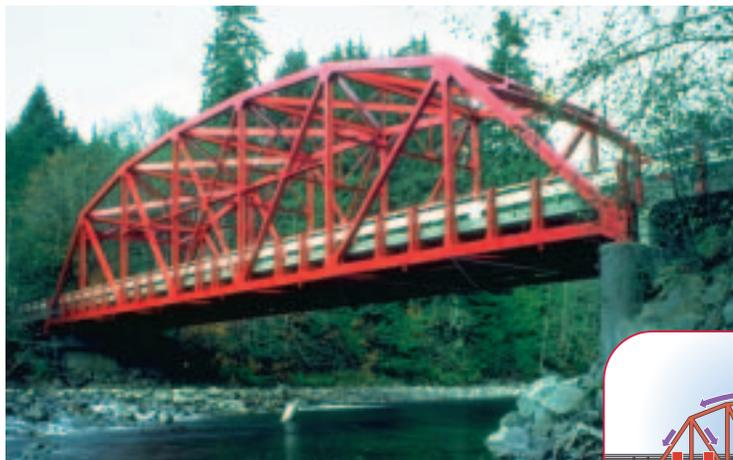
**Figure 2.16** A truss bridge
